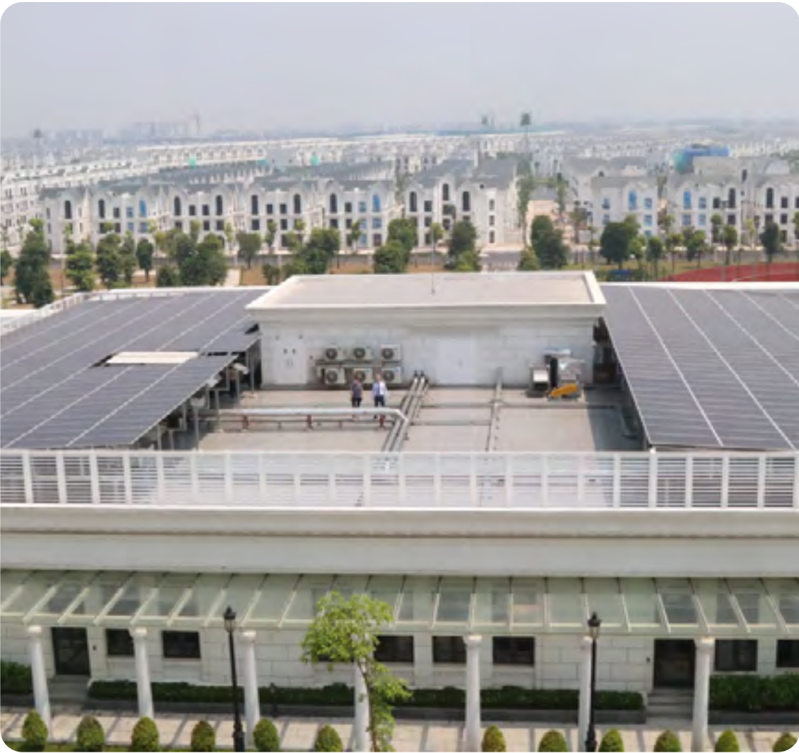
In the Pillar C, VinUniversity installed a rooftop solar power system with a total area of 1,000 m 2 , providing an average of 600kWh per day, and producing more than 163,800 kWh of energy in total.
